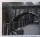
Frederick Pelham designed the stone bridge over Mill Creek in Dexter, Michigan. American Bridge Historical Society
